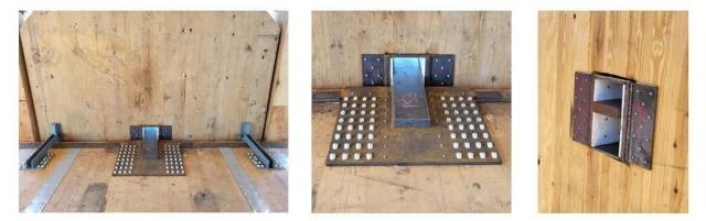
Left: Slotted shear key connection overview; Middle: Closeup view of fasteners; Right: Back side of shear key
