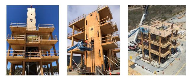
Left: Placing the south rocking wall; Middle: Site staff installing temporary post-tensioning; Right: First three stories complete
