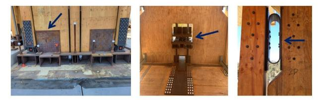
Left: Rocking wall with base shoes; Middle: Temporary post-tensioning for construction bracing; Right: UFP between wall panel and bounding column
